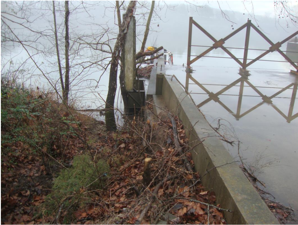
Photo 19 – Typical Steel and Concrete Temporary Barriers
