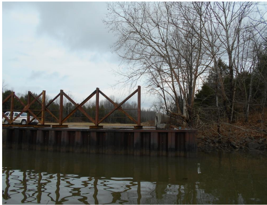
Photo 2: Z Sheet pile wall (northeast corner)
