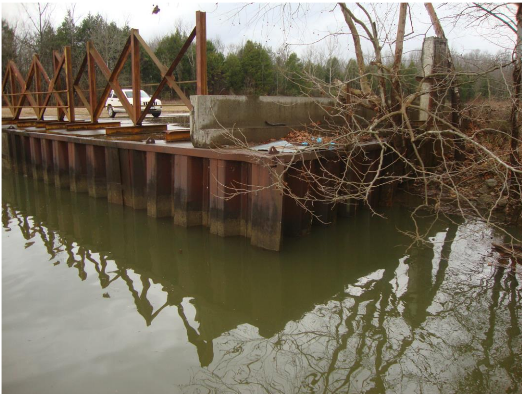
Photo 18 – Typical Steel and Concrete Temporary Barriers
