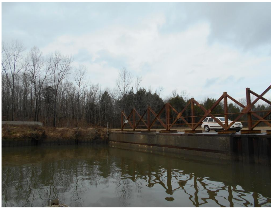
Photo 4: Concrete cap over Z- sheet pile wall
